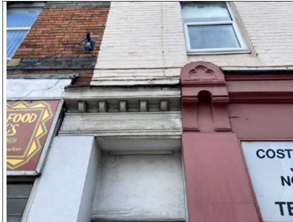
Dentil and corbel features to the left of the shopfront and over door to upper floors. Timber box hoardings covering pilasters.
