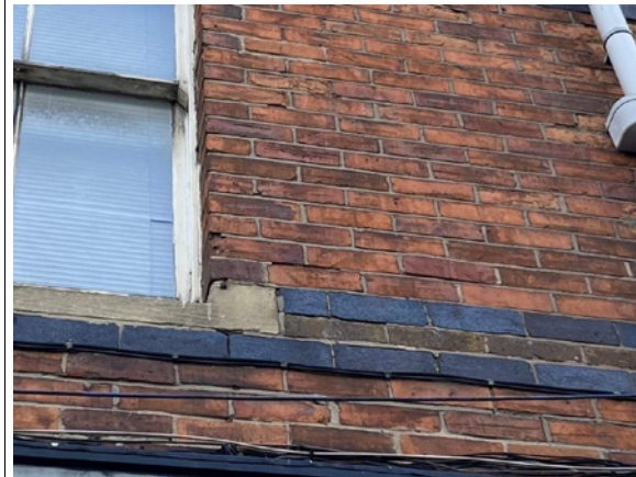
Condition of brickwork on upper levels façade.
