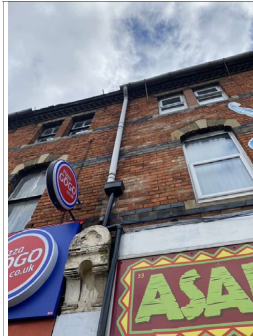
Patch repairs to brickwork visible on upper floors.
