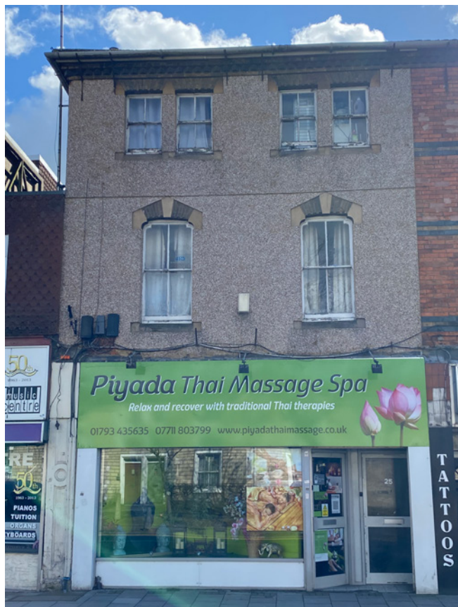
No.25 Faringdon Road. One of the most altered façades, having a modern shopfront, aluminium door to the upper floors and rendered upper floors.
