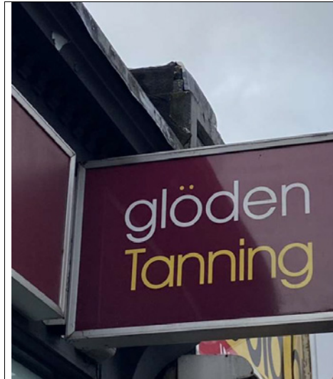
Aluminium box signs to fascia and projecting sign.
