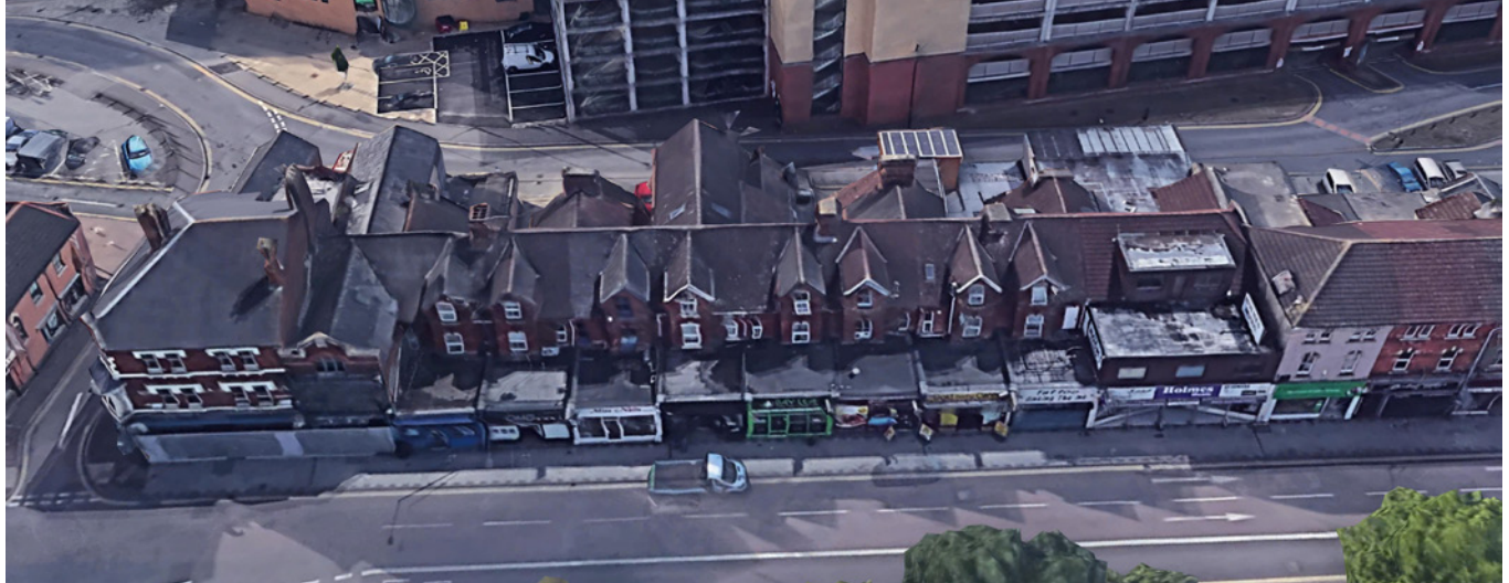
The eastern terrace (5–23 Faringdon Road) © GoogleEarth 2022
