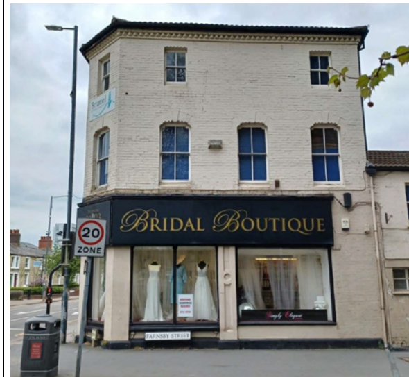
Return elevation to Farnsby Street
