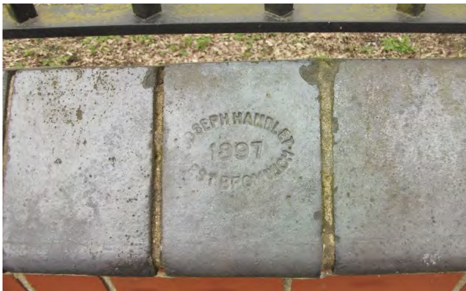
Figure 2.13: A number of the 'blue' coping stones to the boundary wall are stamped Joseph Hamblet, West Bromwich, 1897.
