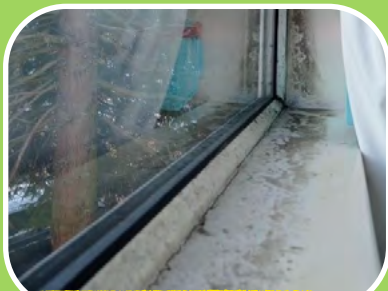
Dark mould around PVC or Windows
