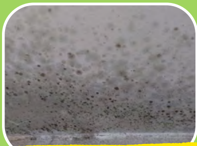
Mould at wall / floor junction
