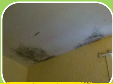
Mould on ceiling
