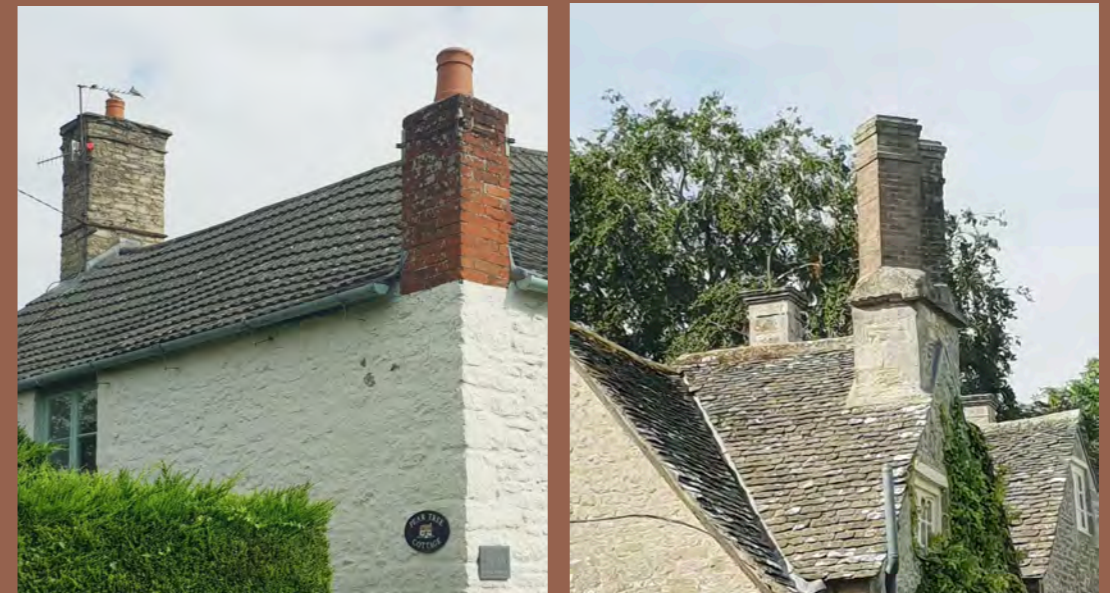
FIG 22 BRICK AND STONE CHIMNEYS
