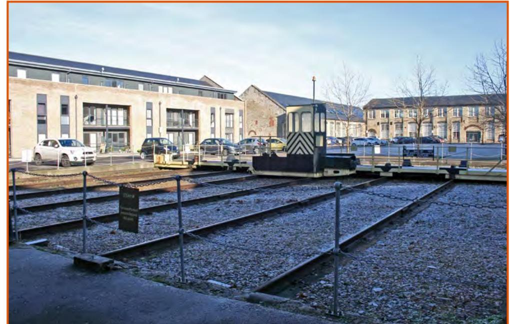
**Fig. 20:** The 1950s traversing table is an example of the visible, archaeological remains from railway works
