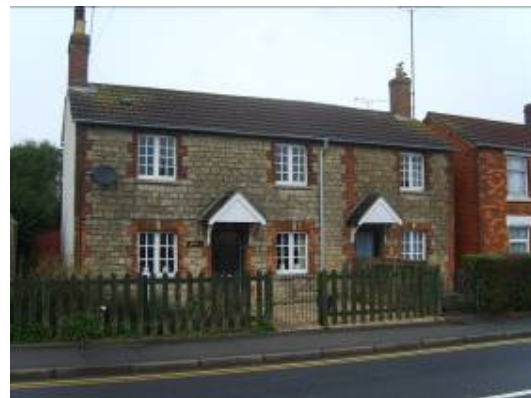
Nos. 3/5 Kingsdown Road, a good example of a pair of 19 th century workers' cottages.
