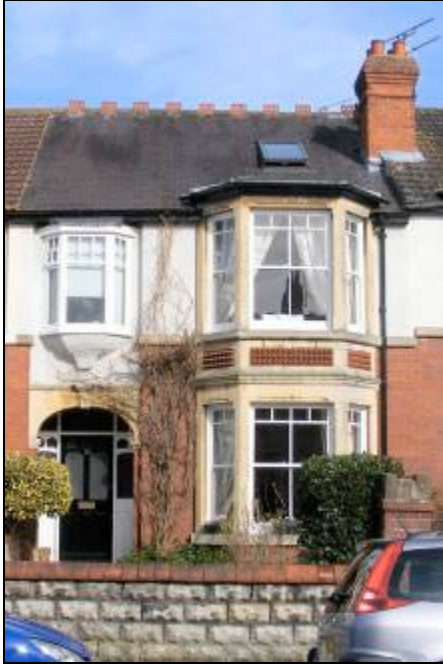
Photograph 3 A typical house-type retaining original features, including timber sash windows, Welsh slate roof and open porch.
