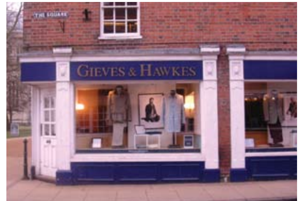
Fig 11. Traditionally detailed stall riser and door
