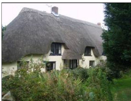
Typical eyebrow dormers in a thatched roof.
