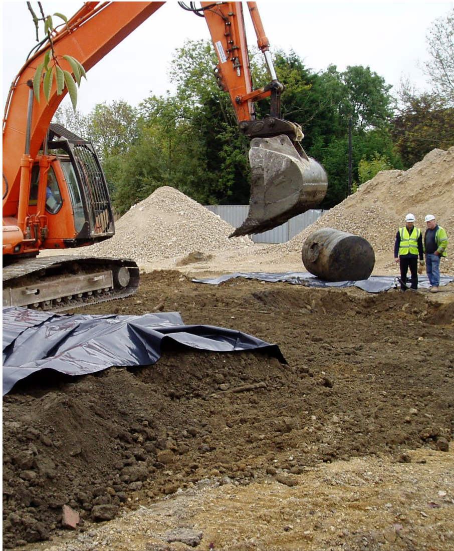
FIGURE 1 Removal of disused underground fuel tanks
