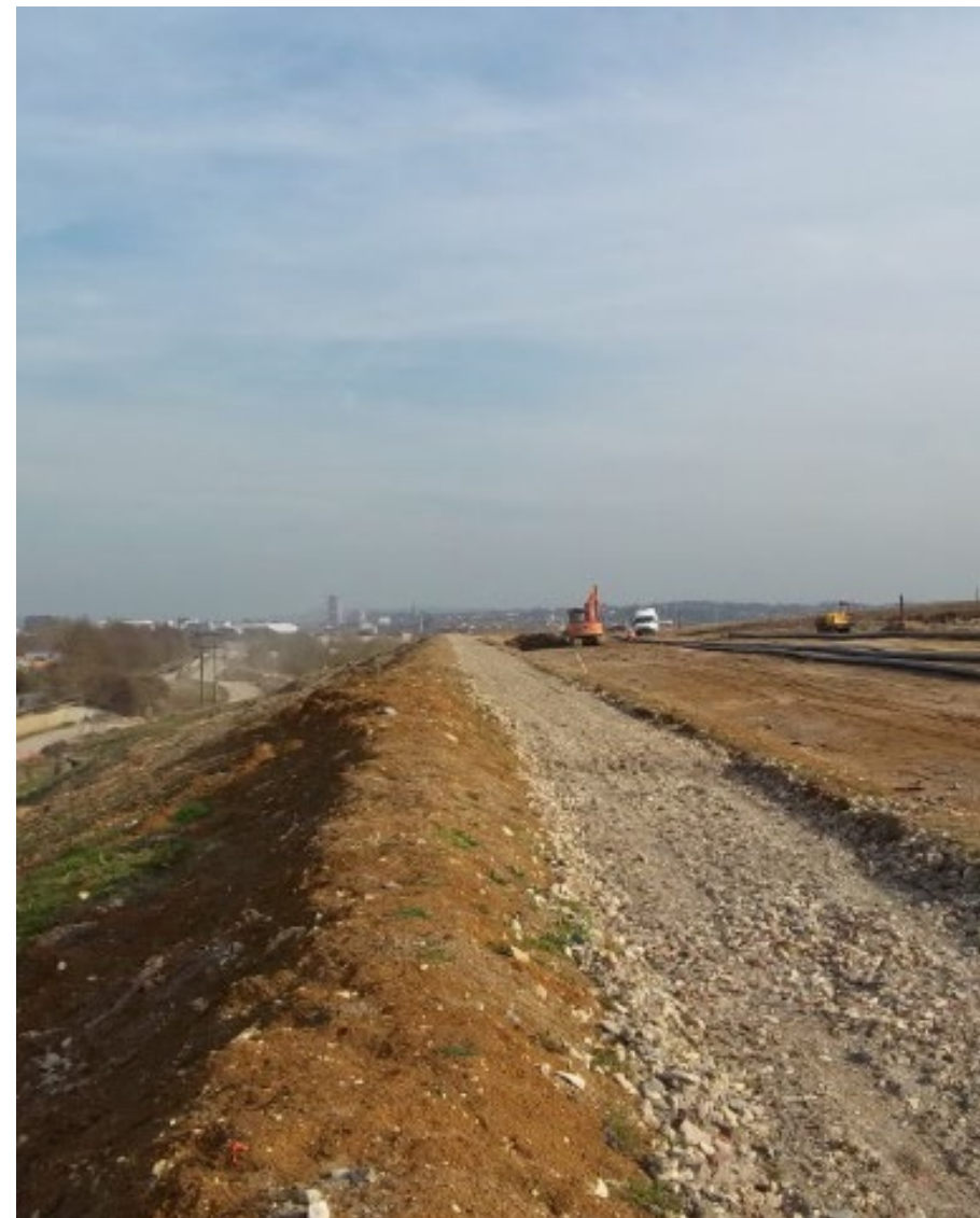
FIGURE 11 Shaw Landfill Site Restoration works by SBC
