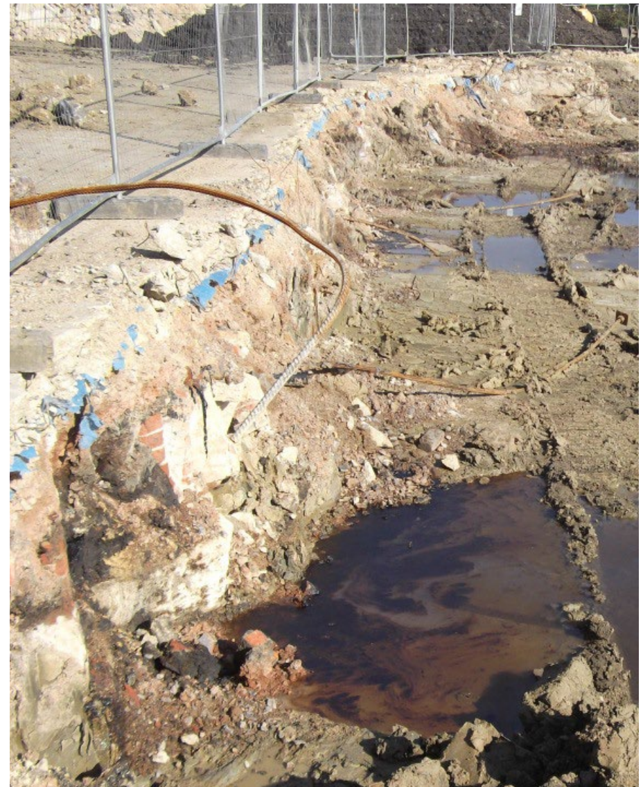
FIGURE 12 Oil Contamination of groundwater
