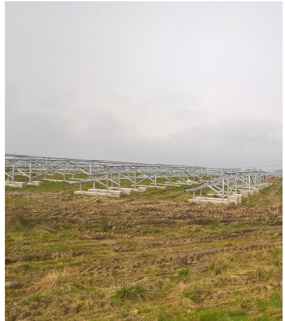
FIGURE 14 Shaw Farm Landfill Solar installation
