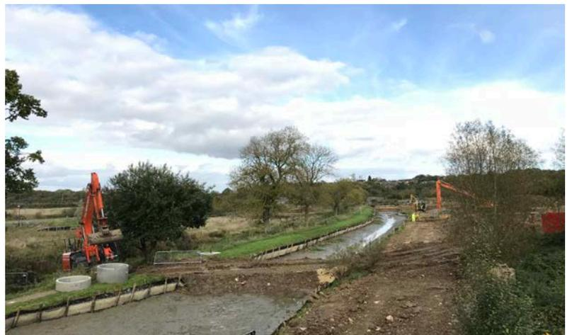
The water has been pumped to both the north and the south so that we can fill the section back up once the works are done. All the fish (including one rather large one) were caught under ecological supervision and moved into the adjoining sections.
