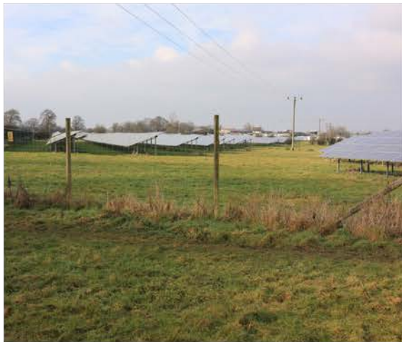
Solar farm north of Wroughton
