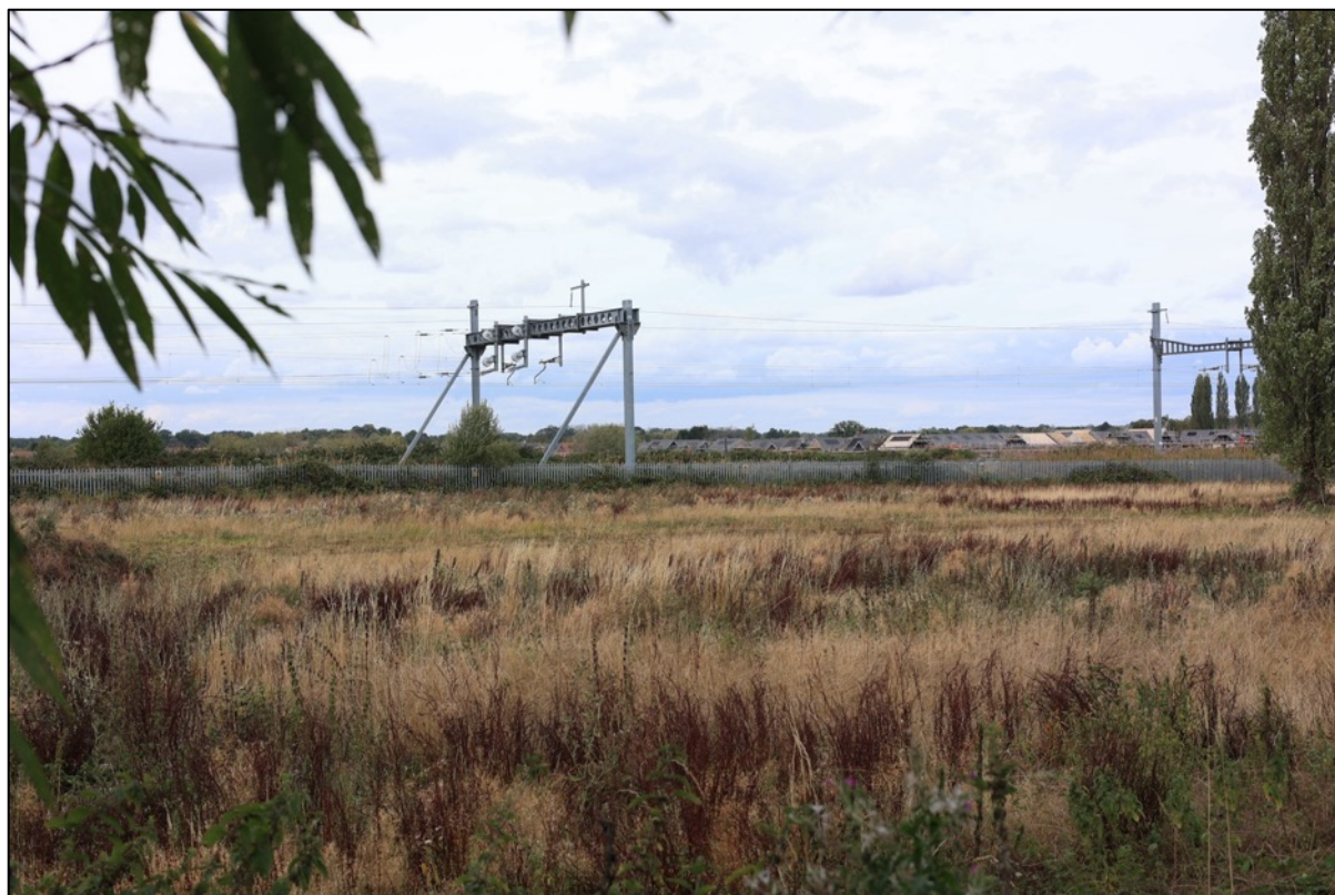
Site 13: View across rough grassland towards the railway corridor, with overhead line equipment, security fencing and development beyond forming prominent man-made influences.
