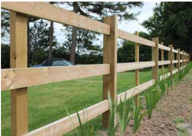
MORTICED POST AND RAIL FENCE
