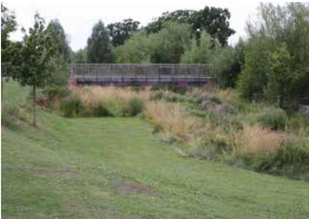
ATTENUATION FEATURE WITH FOOTBRIDGE CROSSING
