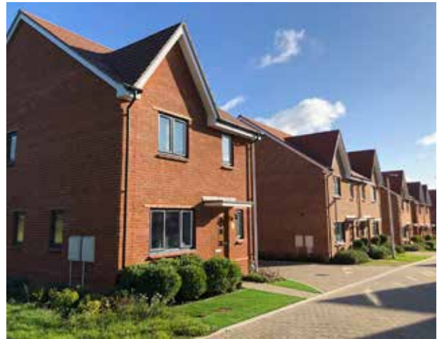
A COMBINATION OF SEMI-DETACHED AND DETACHED DWELLINGS WITH GABLE FEATURES
