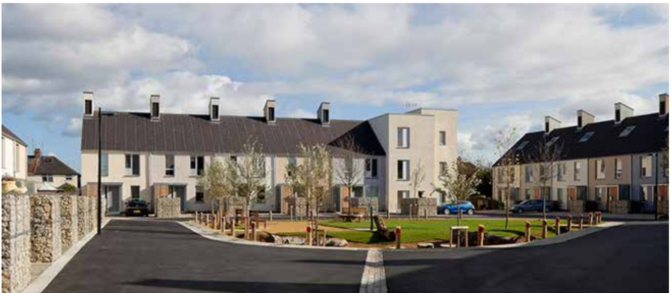
EXAMPLE OF SUDS FEATURES AT "THE TRIANGLE" SITE IN SWINDON
