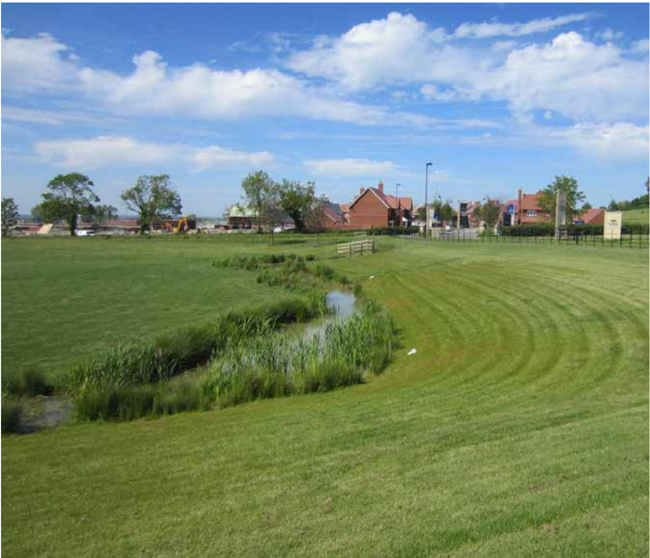
ATTENUATION BASIN WITH SHALLOW SIDE SLOPES
