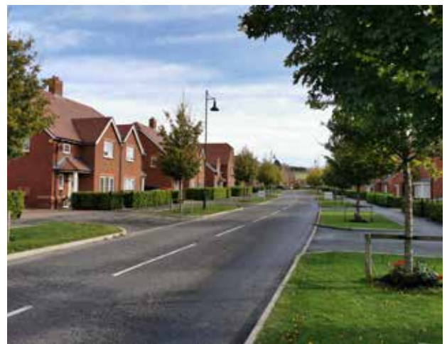
PRIMARY STREET PLANTING REFERENCE IMAGE: VERGES WITH ESTATE RAILING AND HEDGE FRONTAGES
