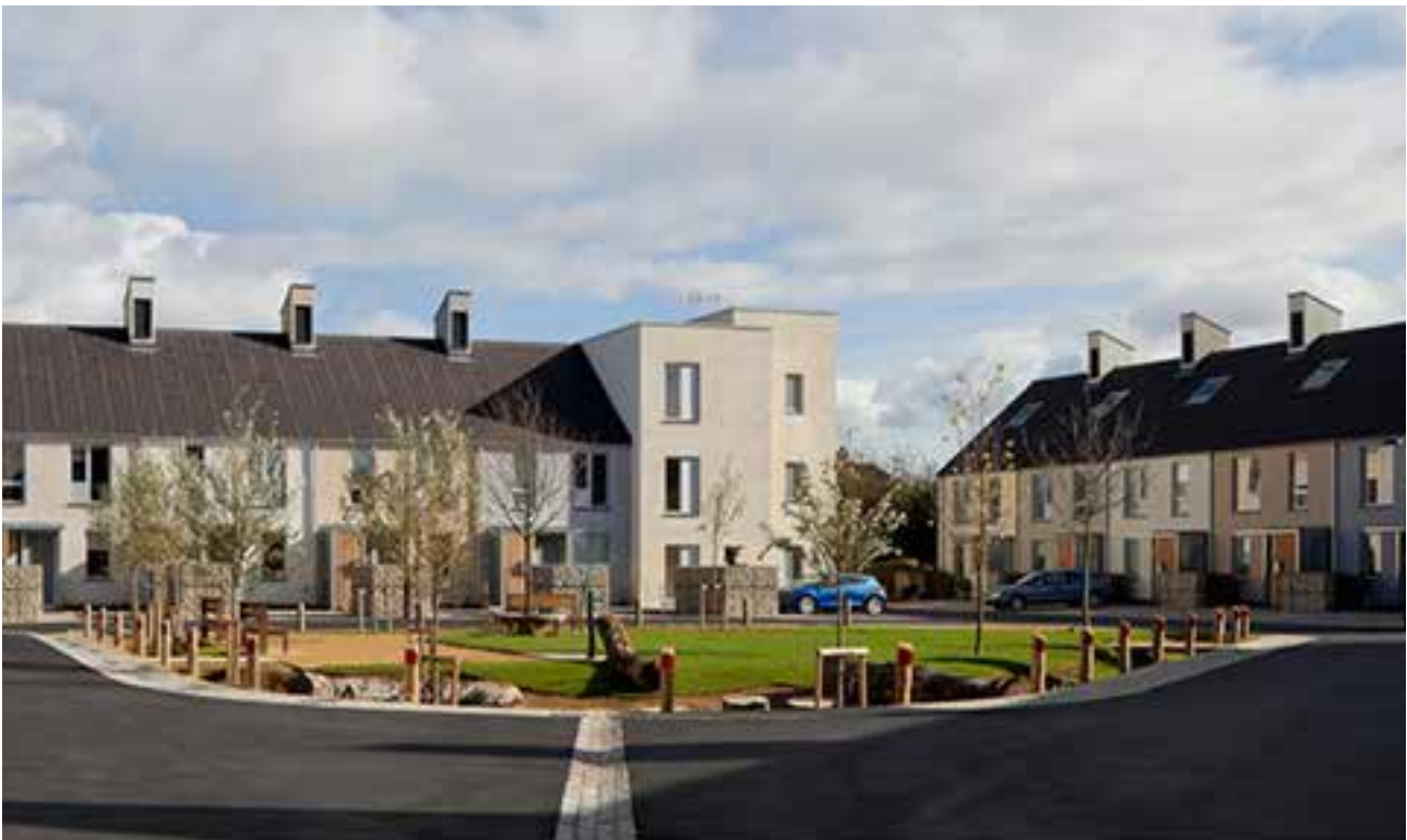
EXAMPLE OF SUDS FEATURES AT "THE TRIANGLE" SITE IN SWINDON
