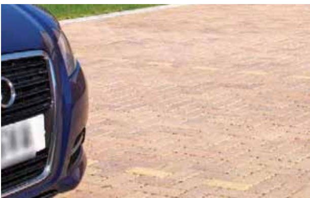
PARKING SPACE WILL BE DELINEATED BY A SUBTLE COLOUR CHANGE TO INDIVIDUAL BLOCKS
