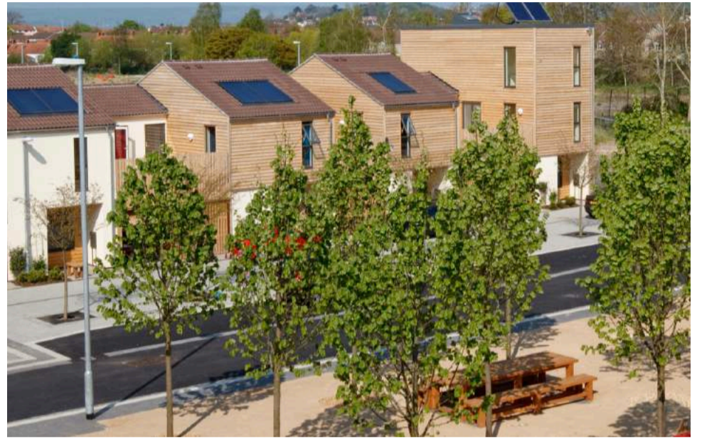
EXAMPLE OF PEOPLE-FRIENDLY PUBLIC REALM DESIGN THAT AVOIDS VEHICLES DOMINATING THE SPACE
