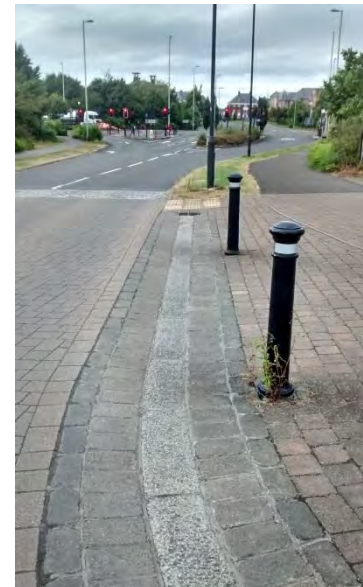
Figure 28 Over the edge paved swale
