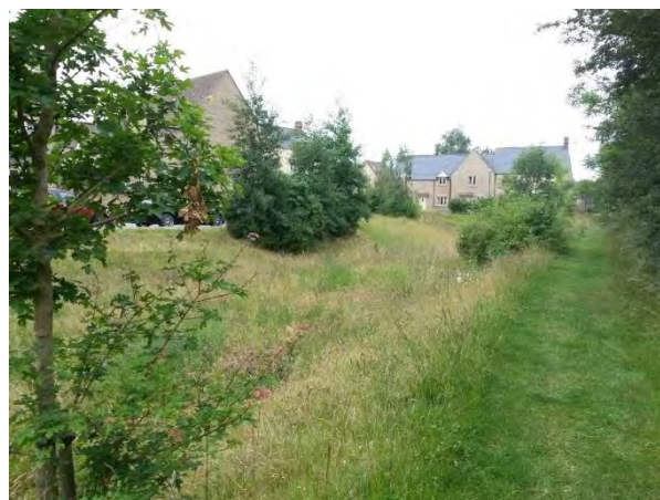
Figure 43 Regional scale detention basin providing visual amenity, water quality and biodiversity benefits, with public right of way along bank area.
