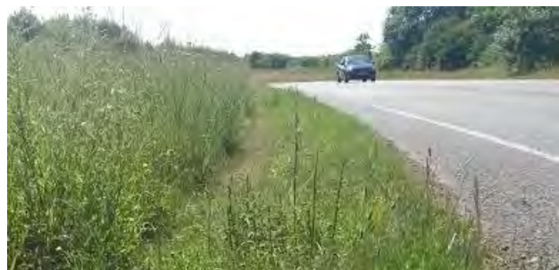
Figure 32 Over the edge drainage on a soft verge
