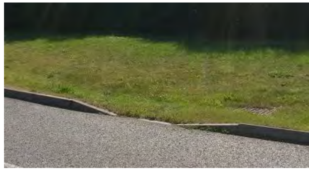
Figure 31 Use of drop kerb to provide inlet
