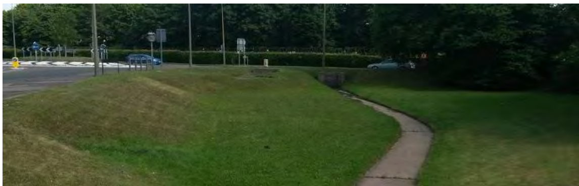
Figure 34 Example of regional scale swale with concrete channel, gradually sloped for ease of maintenance and visual amenity benefit.
