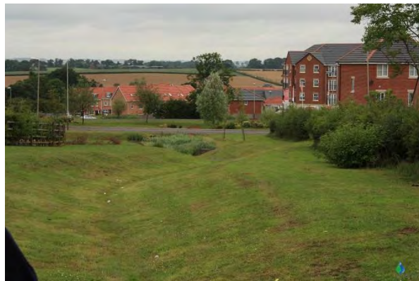
Figure 2 SuDS swale forming soft boundary of new development (courtesy of SUSDRAIN and CIRIA)
