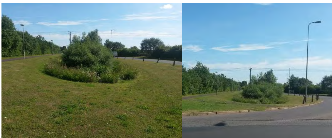
Figure 35 Example of roadside bio-retention cell providing biodiversity benefits.
