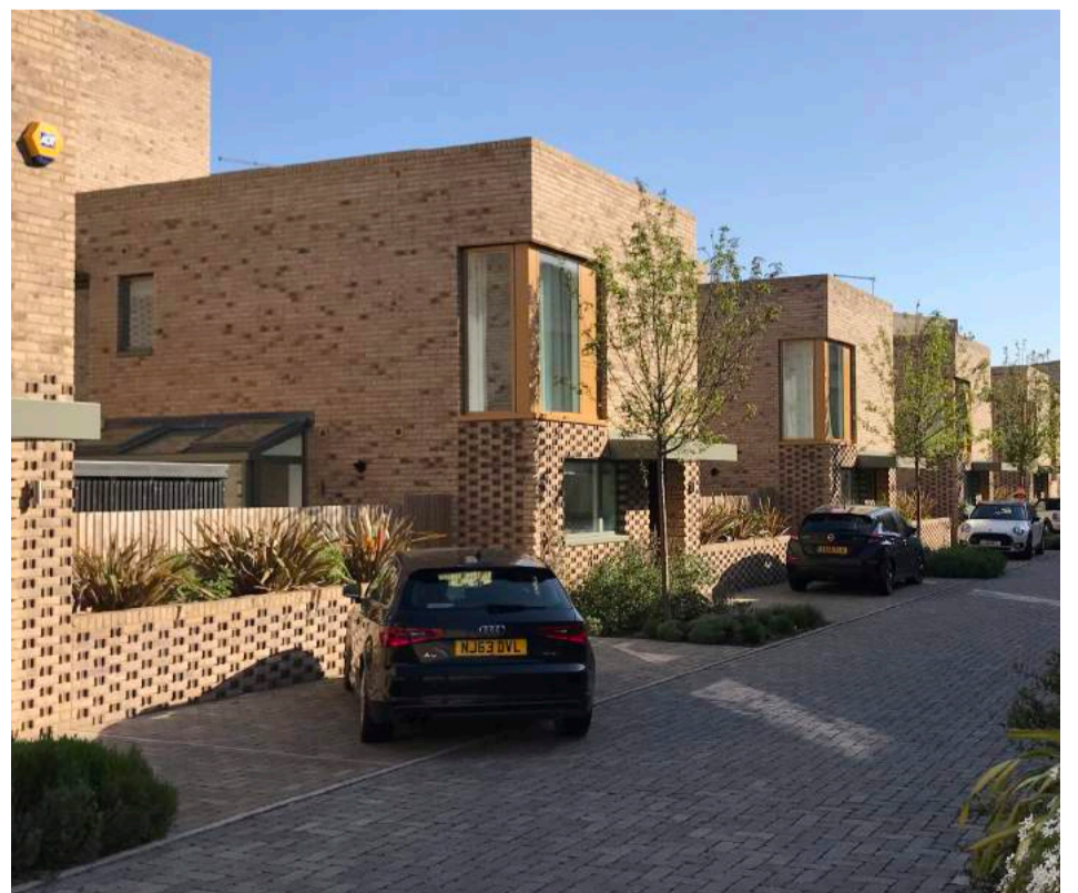
A SUBTLE CHANGE IN SURFACE MATERIAL DEMARCATES IN-CURTILAGE PARKING PUNCTUATED BY TREE PLANTING AND SOFT LANDSCAPING
