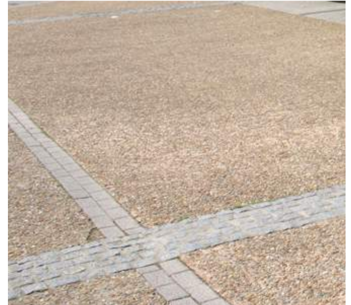
SUBTLE CHANGE OF MATERIAL USED TO DEMARCAT CAR PARKING
