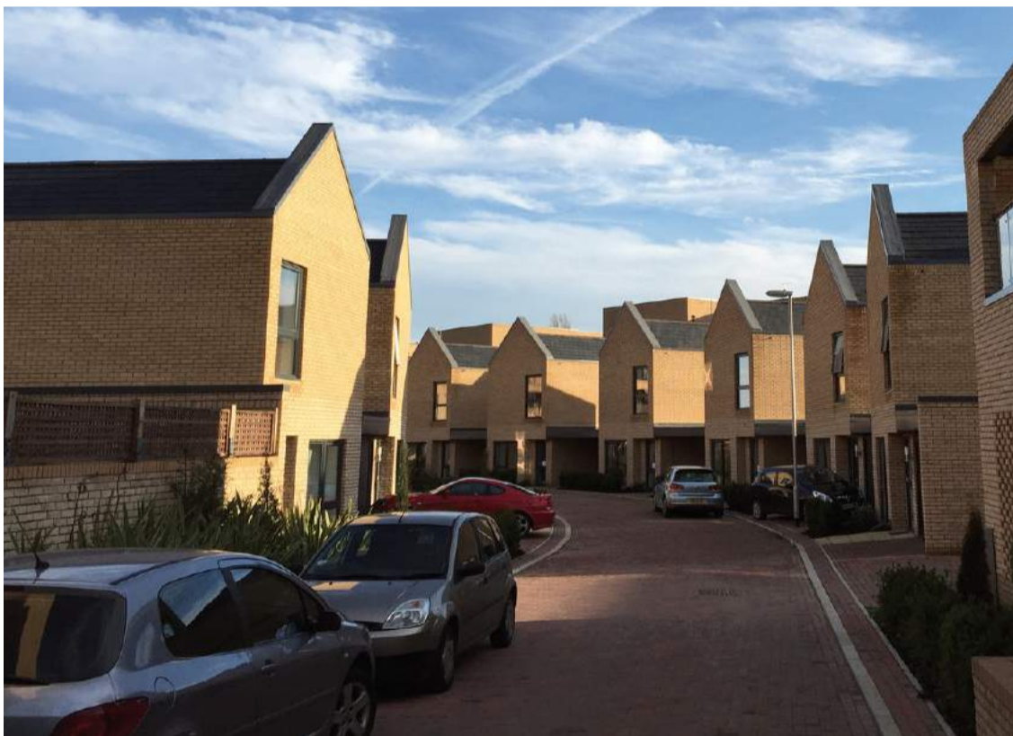
EXAMPLE OF INSUFFICIENT SPACE RESULT IN CARS PARKED WITHIN THE CARRIAGEWAY
