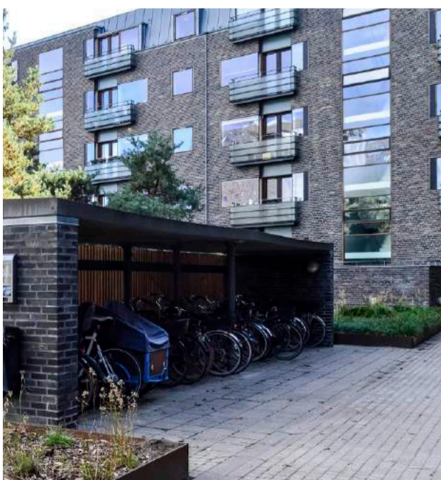
EXAMPLE OF LACK OF LIGHTING WITHIN THIS CYCLE STORAGE AREA
