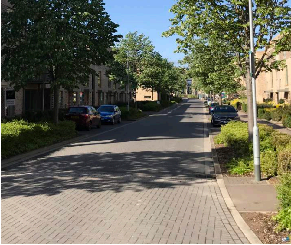
RAISED JUNCTIONS PROVIDE TRAFFIC CALMING MEASURES WHEN APPROACHING RESIDENTIAL NEIGHBOURHOODS
