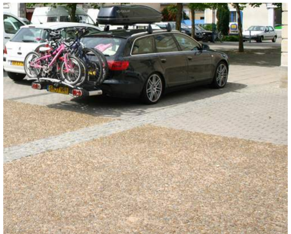
CHANGE OF SURFACE AND TEXTURE DEMARCATES THE CAR PARKING SPACES
