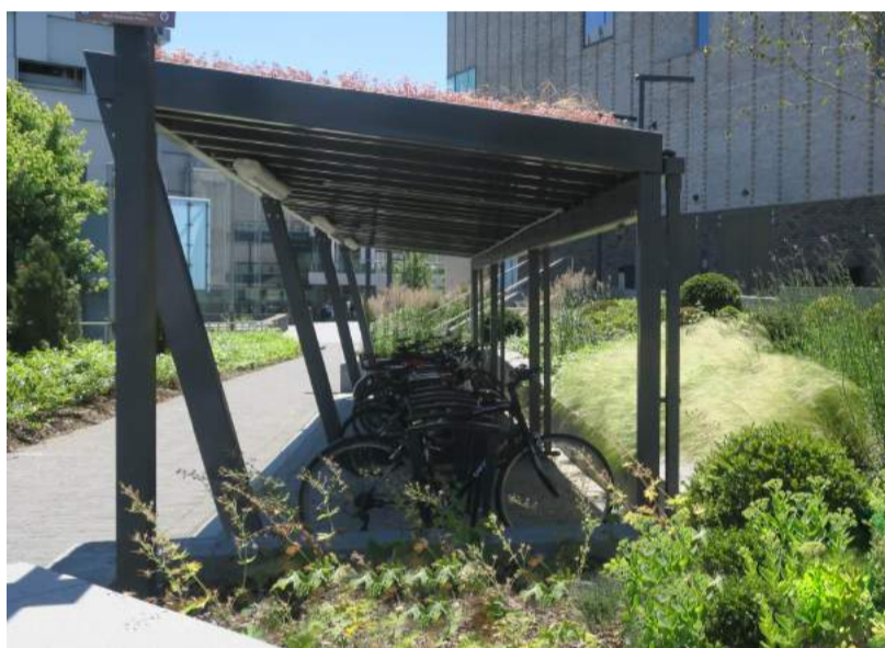
SHELTERED AND OVERLOOKED CYCLE PARKING FACILITIES
