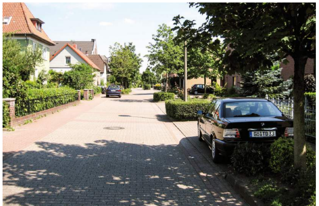
HEDGES, TREES AND HARD SURFACES ARE DESIGNED TO DEFINE THE PARKING AREAS WITHIN THIS STREET
