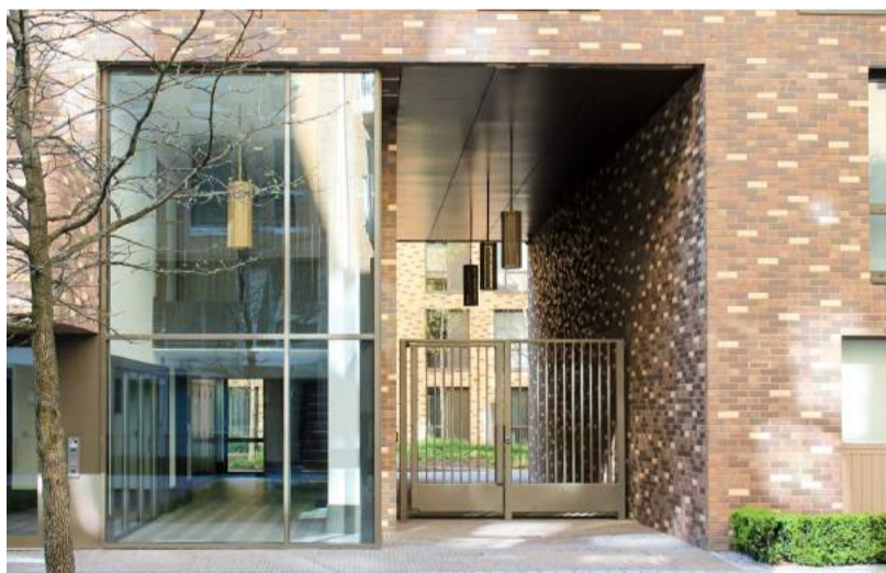
ENTRANCE TO PARKING IS INTEGRATED INTO THE STREET
