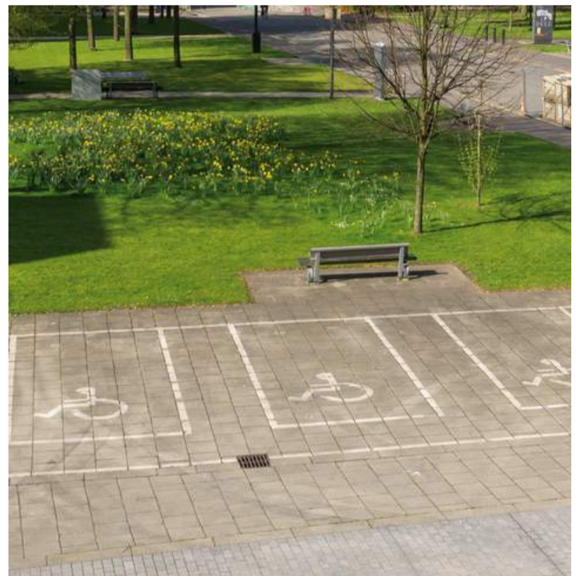
EXAMPLE OF WHITE PAINT IS USED TO DEMARK SPACES
